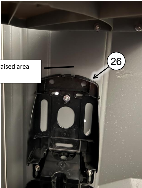
Dispenser installed with (3) 11030 rivets from the outside with 11315 washers on the inside.
