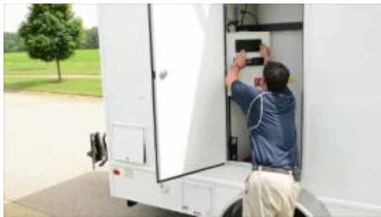
Removing Fuse Panel
