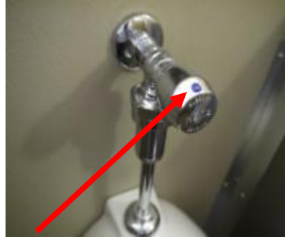
2. Remove Cap and Screw with Allen Wrench.
