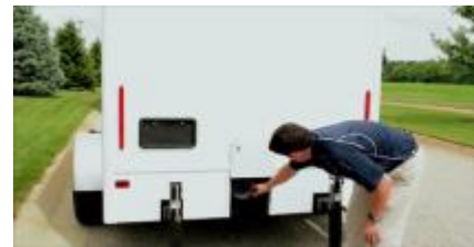
Accessible 4" Clean Out Port.
