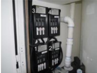
The Satellite Suites™ 25 foot restroom trailer has two to four breaker boxes located in the service area. We suggest checking all breakers you select are in the on position before operation..
