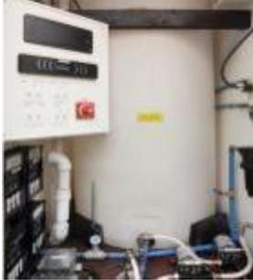
As temperatures fall below freezing your Satellite Suites trailer will need to be winterized, unless it is in operation and equipped with the Arctic Package (see accessories). All water must be removed from the trailer or be treated with RV Antifreeze (propylene glycol). RV Antifreeze is environmentally safe and therefore the only antifreeze recommended for winterizing the trailer.
